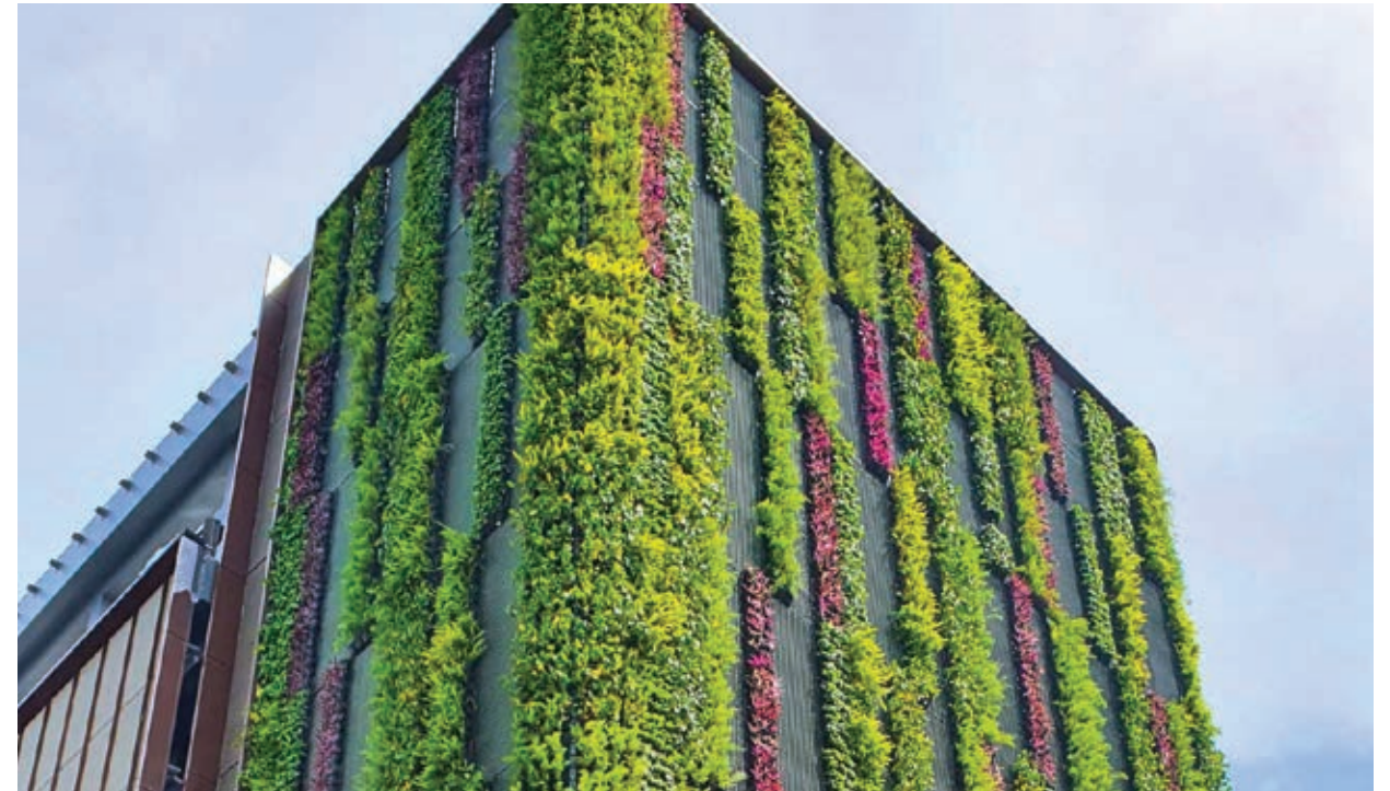
Large-scale vertical greenery installations, such as the 300 m 2 living wall at the National University of Singapore E7 building installed by GWS Living Art, establish vertical garden pockets that weave greenery into the built fabric where horizontal space is scarce. Image: GWS Living Art
