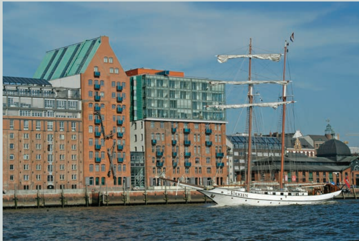
Integration of old and new structures at Holzhafen—with historical warehouses and the Hamburg fish market hall to the right. Image: Christian Spahr, Mediaserver Hamburg
