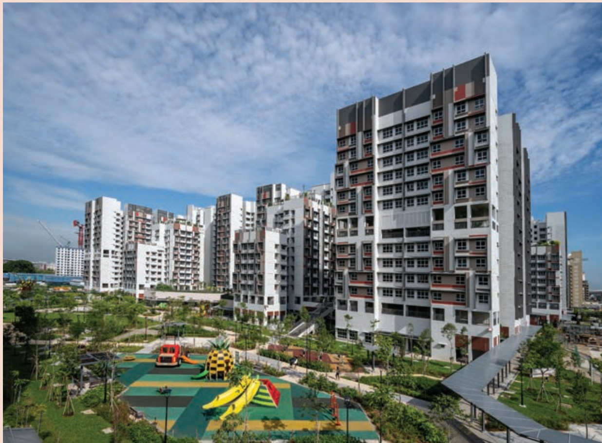
Tengah is designed as a lush evergreen town with car-lite infrastructure, and common spaces spread across the town. Image: Housing & Development Board
