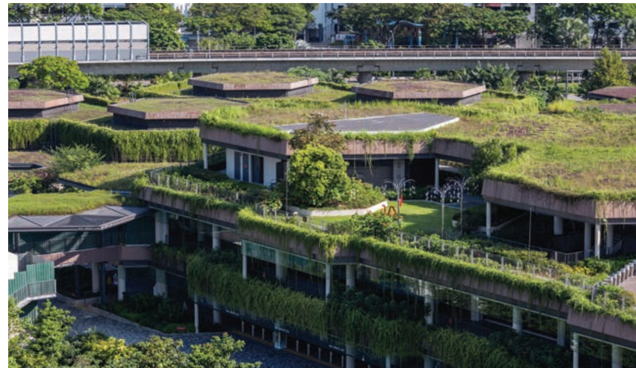
Green roof Gaiamat™ installation at the Sembawang Sports and Community Centre, Bukit Canberra. Green roof was installed by GWS Living Art in 2022 using proprietary, patented, soilless Gaiamat™ that can capture 26 litres of rainwater per square metre. Image: GWS Living Art
